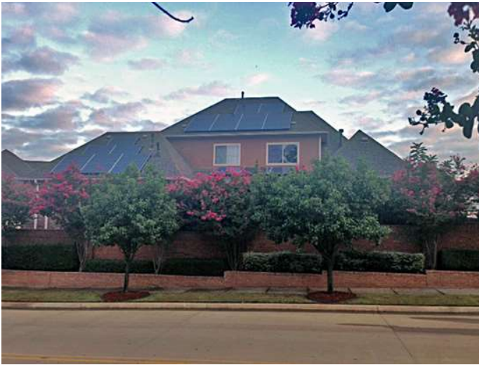
Roof-Mounted SED in Hurst, Texas
