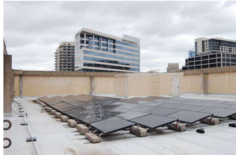
Roof of Oncor Electric building (Dallas, Texas)
